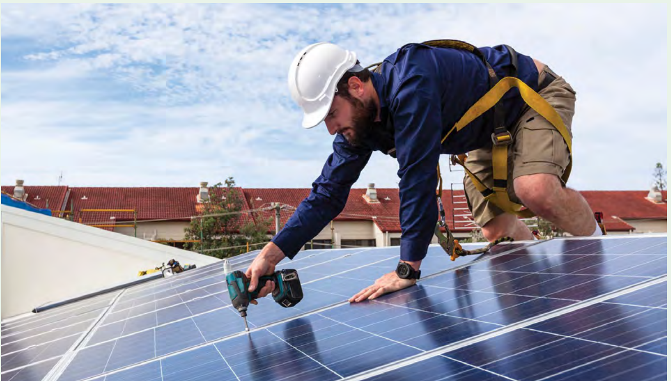
Solar panel technician
