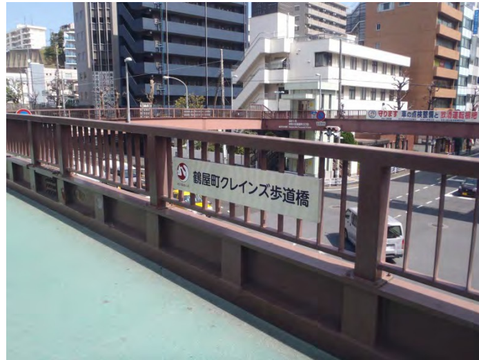
Figure 5-55. Naming rights for road facilities
