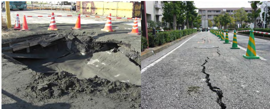
Figure 2-28. Damage in the city after the Great East Japan Earthquake
