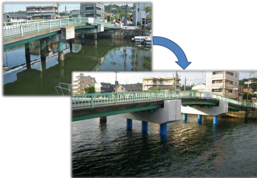
Figure 5-52. Seismic Strengthening of Bridges (Isogo Bridge)
