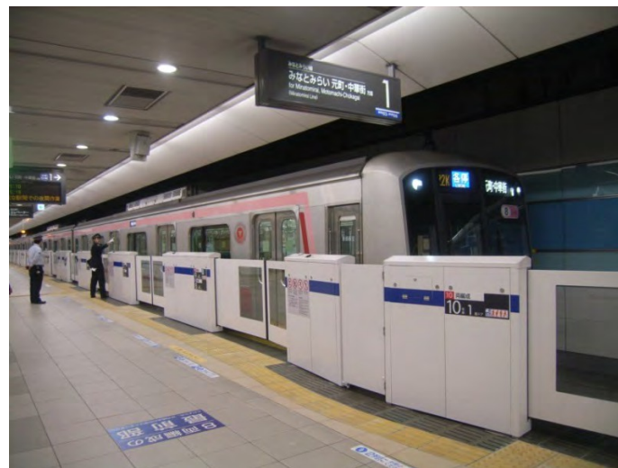
Figure 5-60. Platform Door (Yokohama Station, Minatomirai Line)
