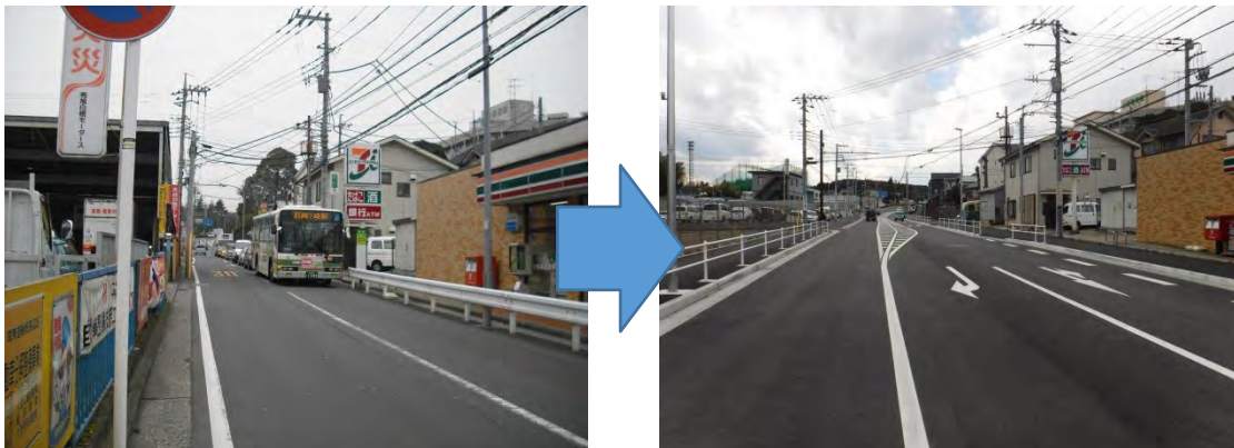
Figure 5-28. Road Widening and Improvement (Asahi Ward)
