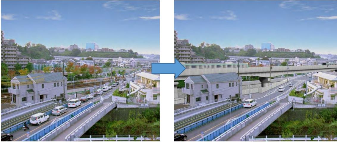
Figure 5-29. Image of the completed continuous railroad intersections project (Sagami Railway Main Line (Hoshikawa - Tennocho Station))
