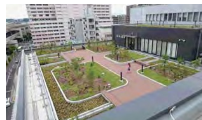
Rooftop greening (Minami Ward Office)
