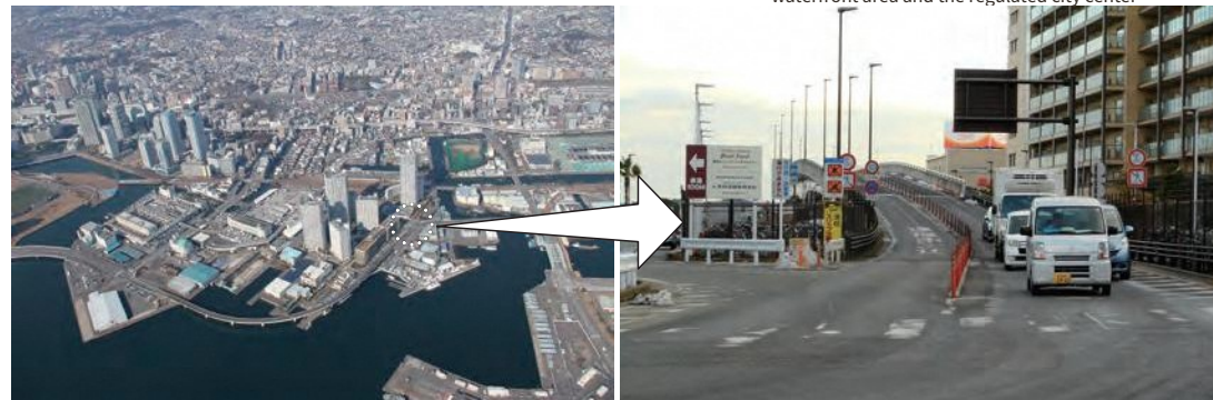
Status of the temporary use section of the Harbor Trunk Highway (Yamauchi Pier)
