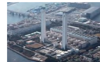
Yokohama Power Station (Courtesy of Tokyo Electric Power Fuel & Power Co.)
