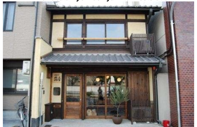
Taniguchi/Cafe Kyo-machiya After Restoration
