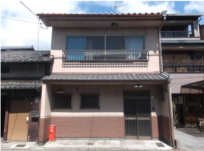
Kawabata Kyo-machiya Before Restoration
