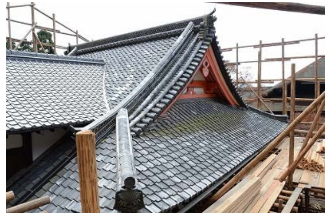
Figure 2.21: Amida Hall Before Overhaul Restoration (Modified Tiled Roof)
