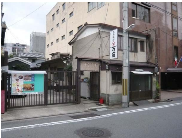
Hachimanyama Kyo-machiya Before Restoration
