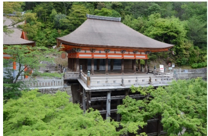
Oku-no-in Exterior – After Restoration
