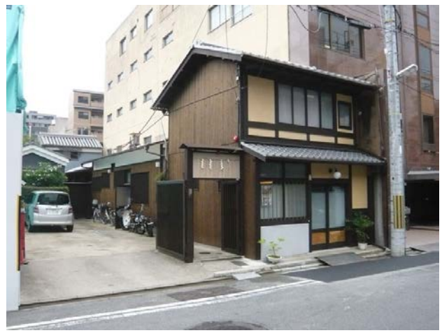
Hachimanyama Kyo-machiya After Restoration
