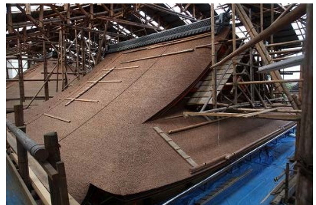
Figure 2.22: Amida Hall After Overhaul Restoration (Original Thatched Roof)
