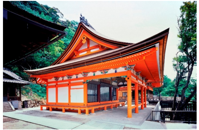
Amida-do Exterior – After Restoration
