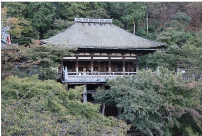
Oku-no-in Exterior – Before Restoration
