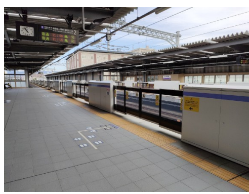
Figure 1. Example of fall prevention platform fence installation (Umekoji Kyoto West Station)
