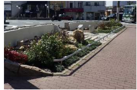
Rain garden developed at the northwest corner of the Kujo Oishibashi intersection
