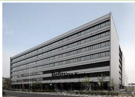
Befitting Kyoto Environmentally friendly buildings (Kyoto City Water Supply and Sewerage Bureau General Office Building)
