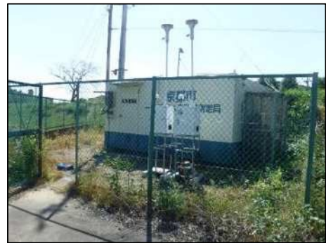
General Environmental Atmospheric Measurement Station
