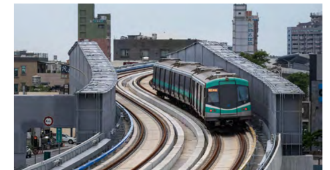
Initial Driving Test of the Gangshan-Luzhu Extension Line (1A Section)
