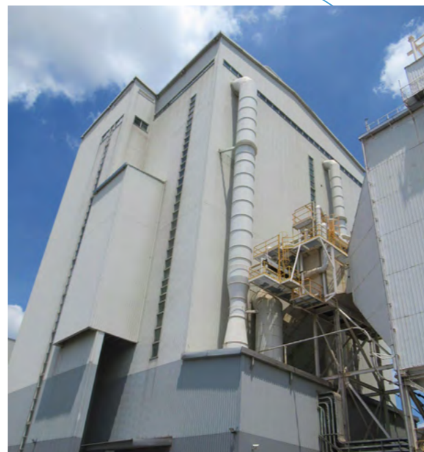
Chung Hwa Pulp's Cogeneration Plant - Largest SRF User in Kaohsiung City
