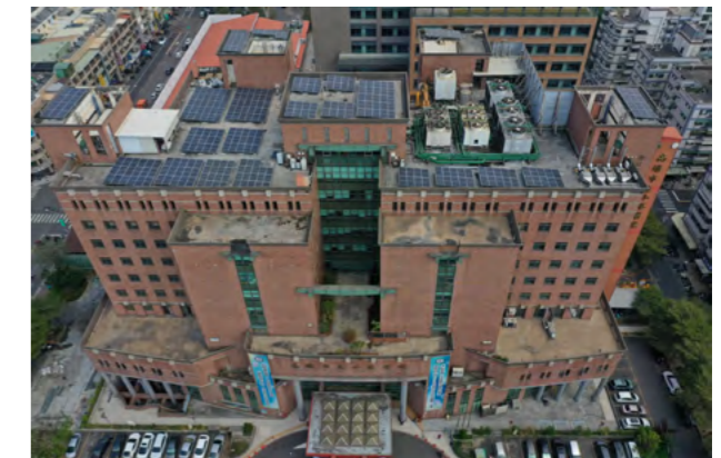
Solar Photovoltaic Installation on Kaohsiung Municipal Siaogang Hospital Rooftop Promoting Energy Diversification
