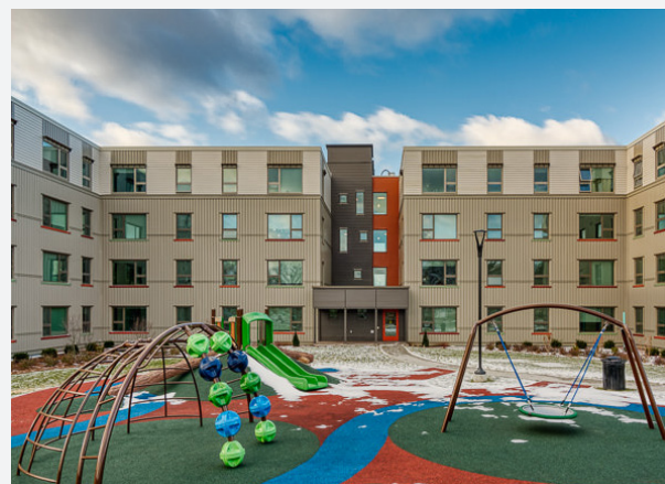
Laurentide, North Avenue, Burlington Vermont Affordable apartments created in partnership with Champlain Housing Trust.
