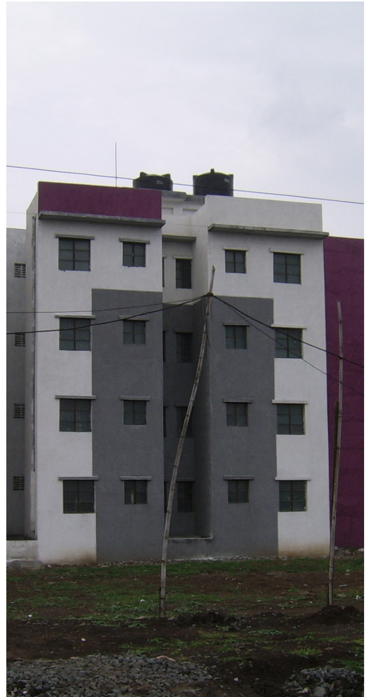
Economically weaker section housing- Surat, Photograph Credit: TARU, India
