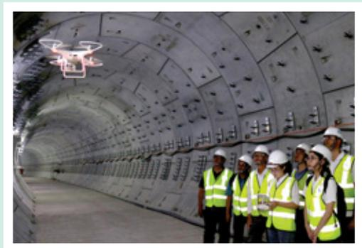
Using drones for tunnel inspections
