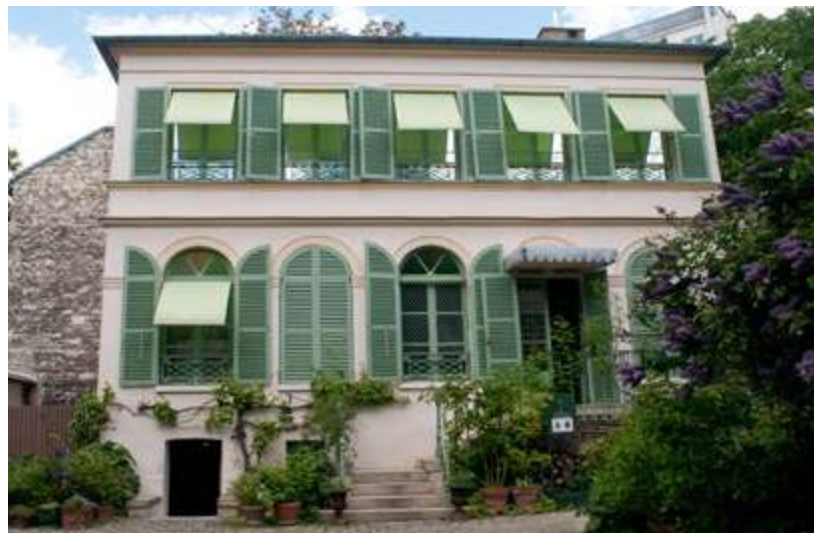
In tandem with these actions, which will be continued in 2022, an Energy Performance Contract (CPE) has been established for the Petit Palais, Cernuschi and Vie Rromantique museums, which have been identified as having the highest energy consumption rates. This contract aims to optimise the output of technical facilities and their management using a transparent investment budget, entirely compensated by the reduction in fluid consumption.
