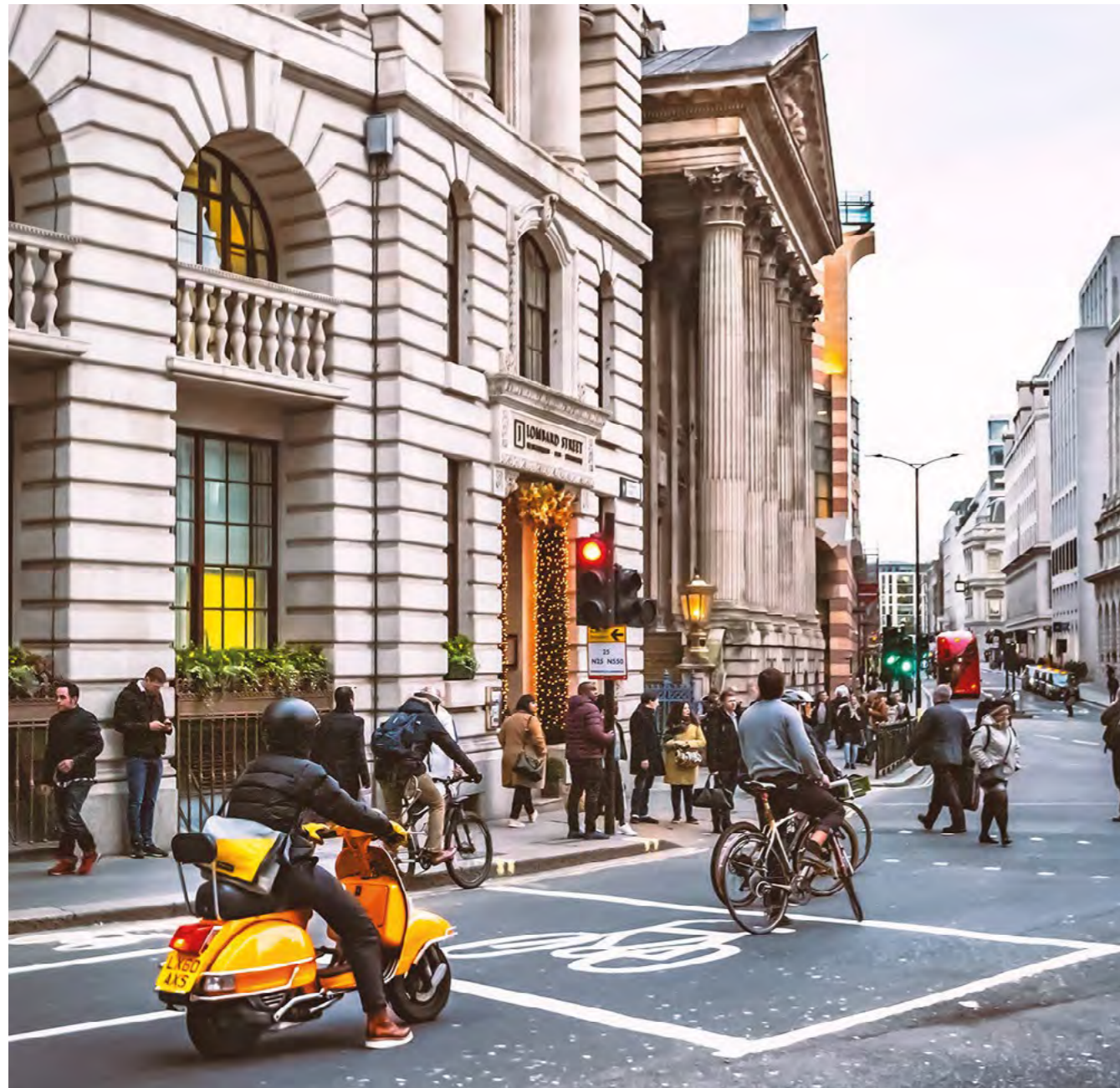
Above: Mansion House
