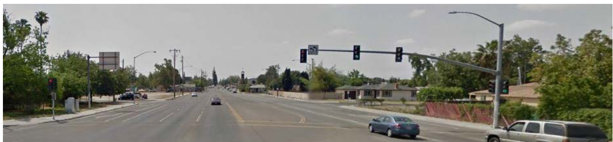
Figure 6: Long crossing (134 feet) at Cedar Ave south of SR 180 (Source: Google Maps)
