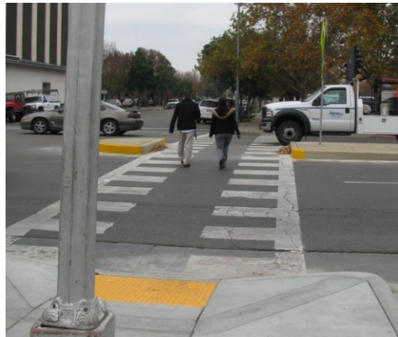
Figure 24: Uncontrolled Crosswalk with High Visibility Markings and Median Refuge Islands in Downtown Fresno
