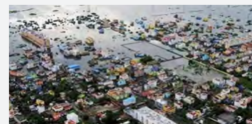
Aerial view of Chennai flooded | Source: PTI
