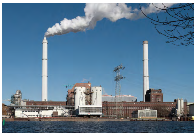
Fig. 19: Power Station Klingenberg in Berlin-Rummelsburg.
