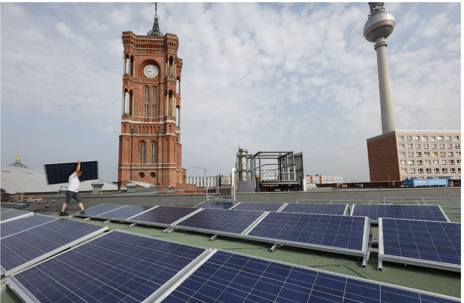
Assembly of the solar roof on the Red City Hall
