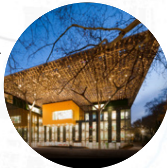
3. Goede Doelen Loterij (Zuidas) Sustainably-renovated office with 'BREEAM Outstanding' quality mark: energy- and water-neutral with PowerWindows and solar panels.
